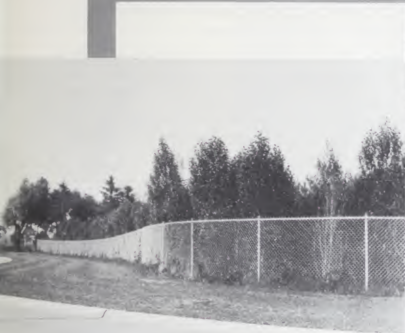
Here is a high Cyclone Safeguard Fence around a park. It not only keeps people from entering when and as they please, but at the same time protects the shrubbery from trampling and breakage. Viewed from the other side such a fence can scarcely be seen through the shrubbery.
